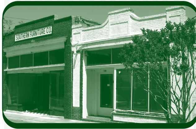
HISTORIC COMMERCIAL PROPERTIES ON NORTH 4TH ST. PROTECTED BY AN EASEMENT.
