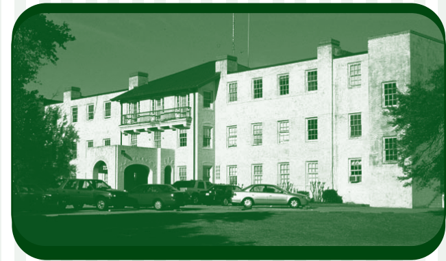
BABIES HOSPITAL WAS LOCATED ON SUMMER REST ROAD IN WILMINGTON. A PRESERVATION EASEMENT WOULD HAVE PRESERVED THIS BUILDING.
