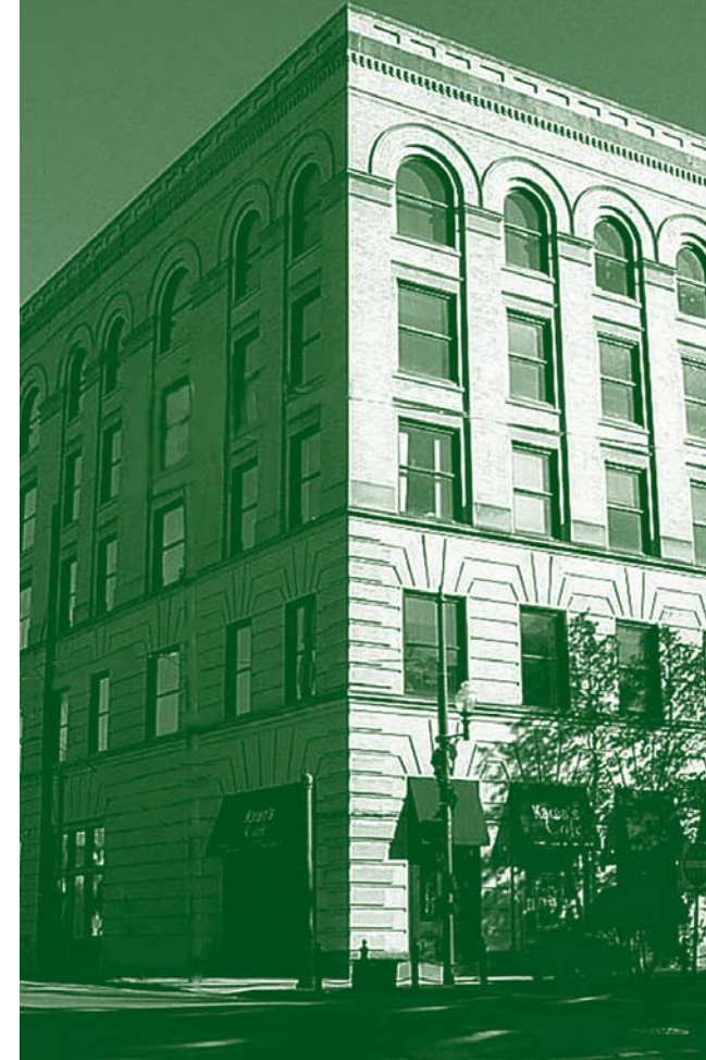
Self Help Center Building, Wilmington, NC
